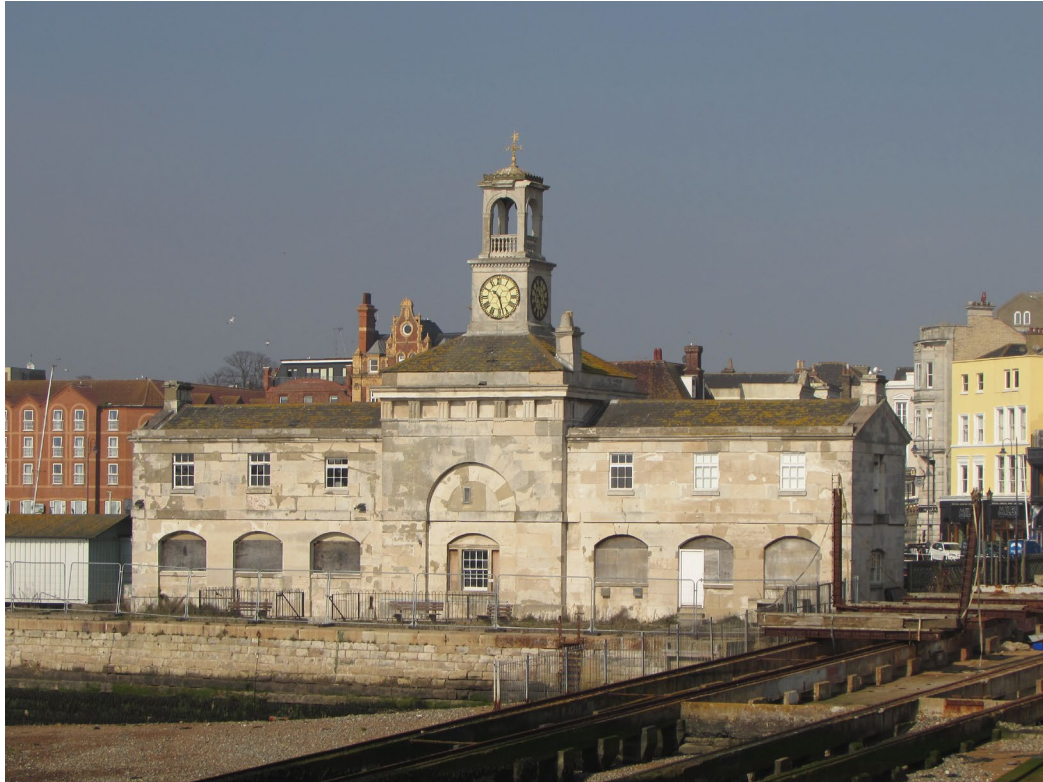
Photograph 4: Southeast-facing elevation of the Harbour Clock House (Listed Grade II*), now Ramsgate Maritime Museum, with slipways in the foreground
